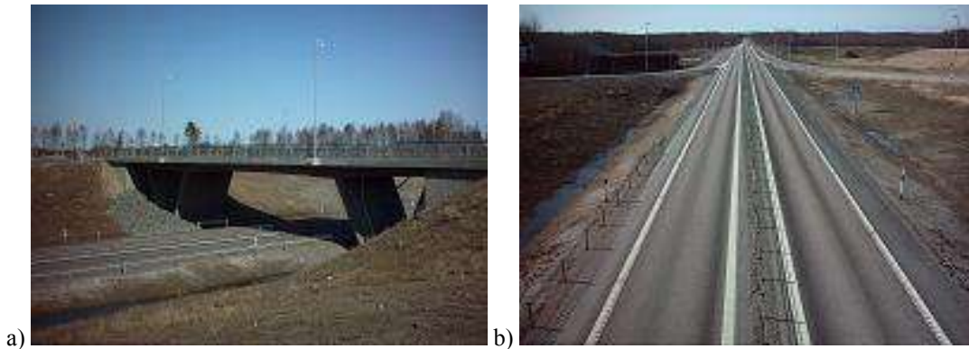
Fig.5.12 a) Junction E4-596 b) View from measure point M E4/596
