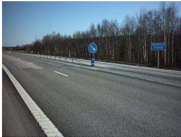
Fig.5.7 Transition from the stretch of road with and without wire rope barriers, Persön
