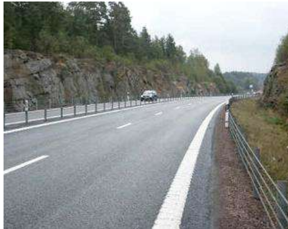
Fig.3.3 Wire rope barrier [17].
