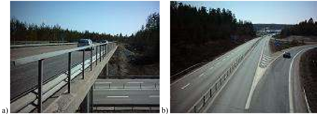
Fig.5.10 a) Junction E4-968 b) View from measure point M E4/968
